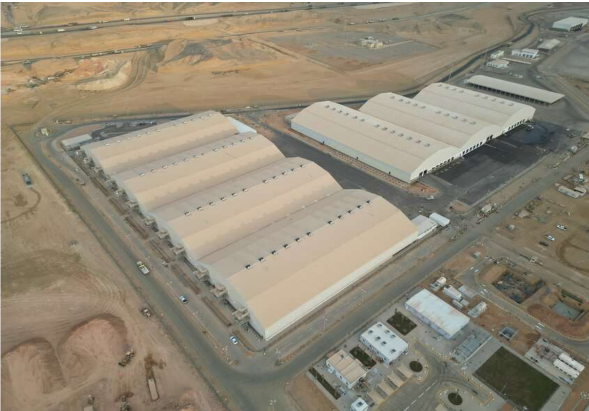
Project Name: NEOM Oxagon Warehouse End User (Client): NEOM Contractor: Al Tamimi Contracting System: Building Management System
